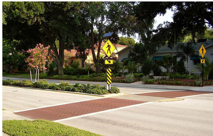
Stamped concrete has the appearance of brick; this both provides a color for visibility and a tactile reminder to drivers to slow down.
