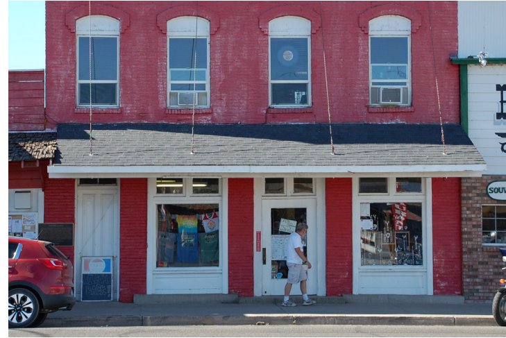
Storefront with canopy
