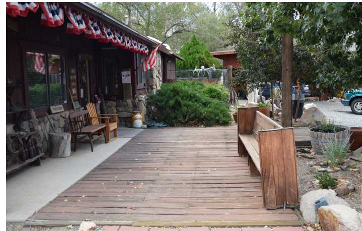
Existing wood-slat walkway runs at the building face, and could extend to an adjoining property to create a pedestrian network.
