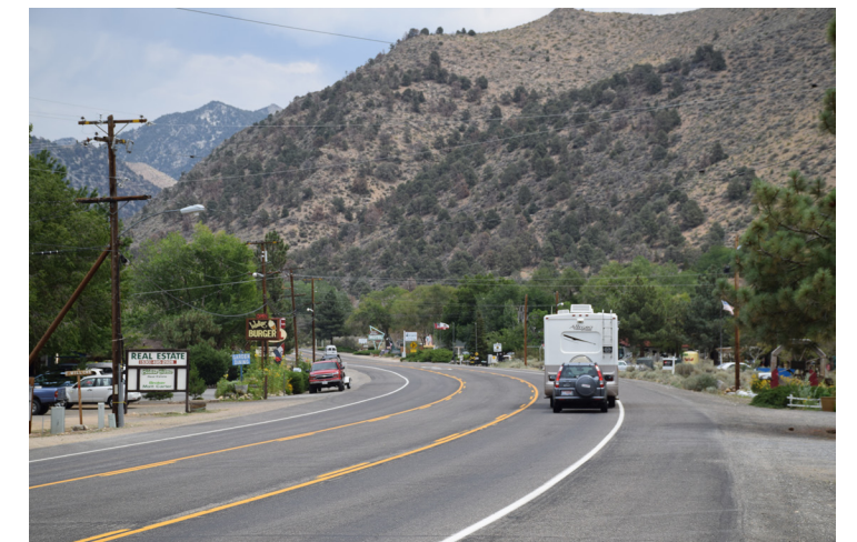
Wide right-of-way encourages high speeds.
