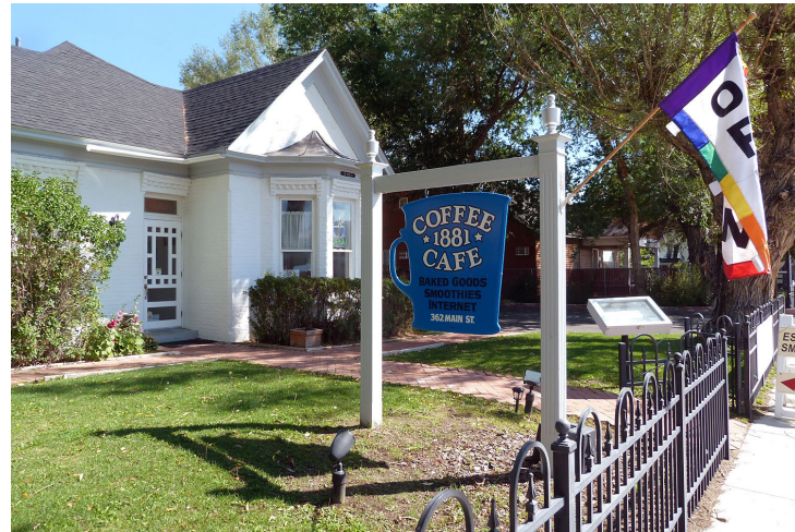
Deep setback with paved walkway and fence
