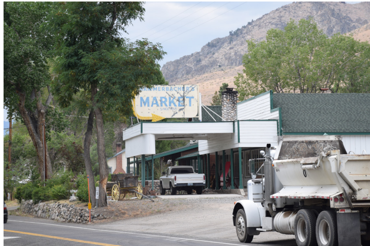
Historic drive-through with retaining wall
