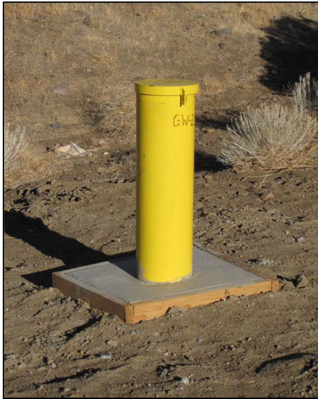
Plate 2-5. LFG monitoring well GW-2 (view NW).
