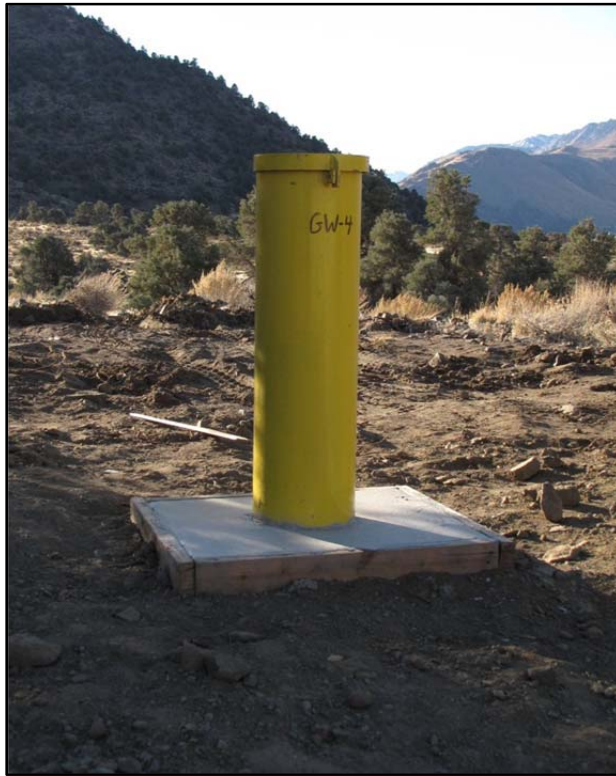
Plate 2-9. LFG monitoring well GW-4 (view south).
