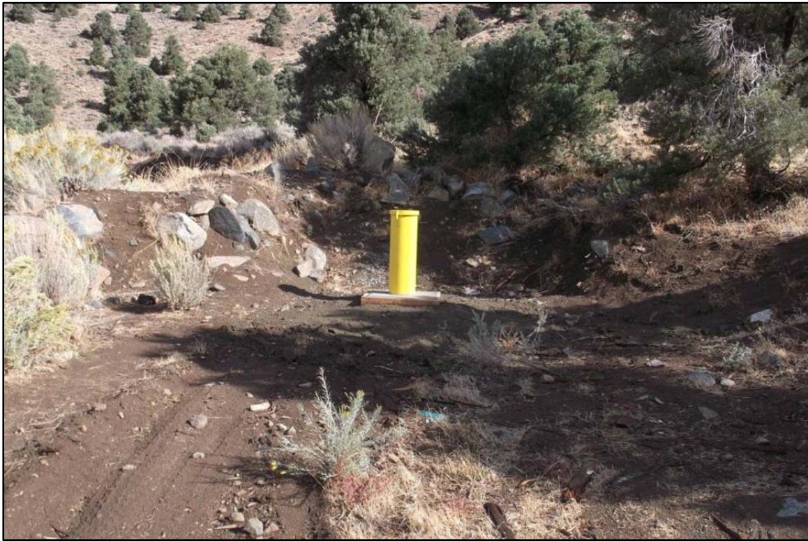
Plate 2-1. Landfill gas monitoring well GW-1 (view north).
