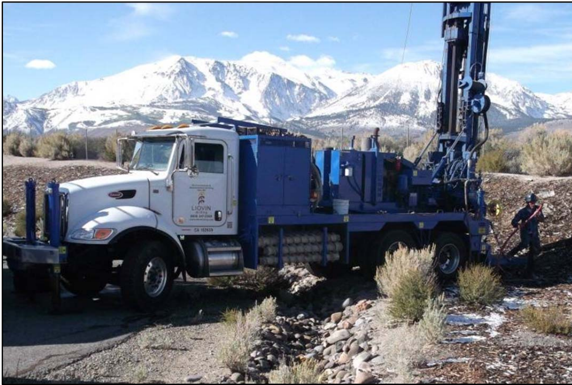
Plate 1-1. Truck-mounted hollow-stem auger rig over borehole (PV LF GW-1, view west).
