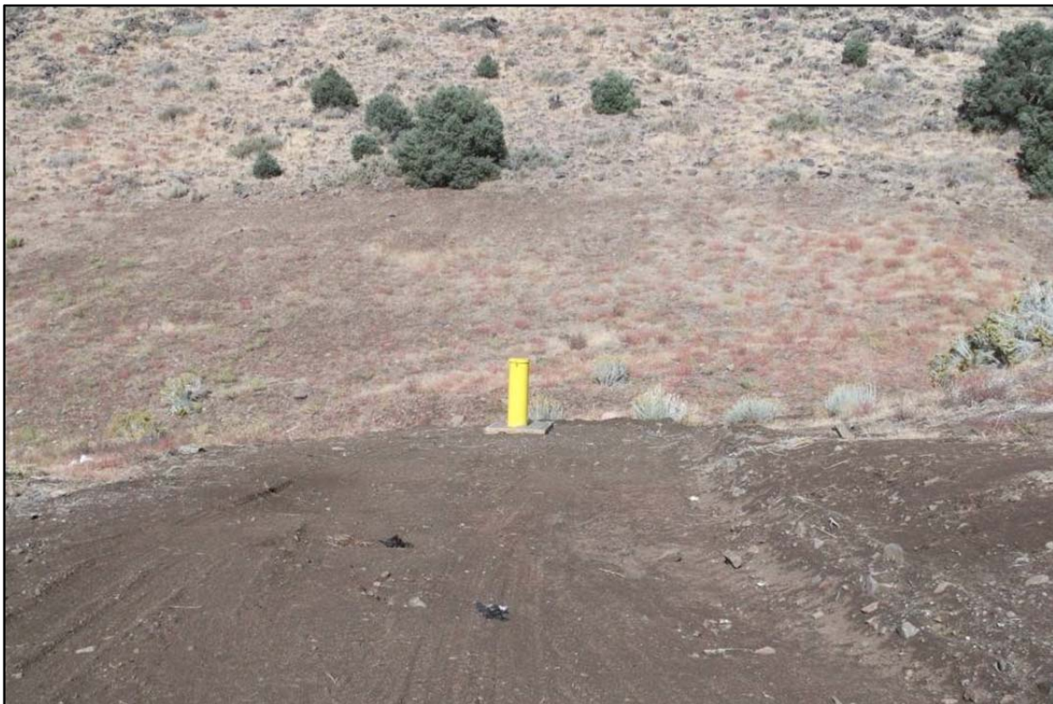
Plate 2-4. Landfill gas monitoring well GW-2 (view west).
