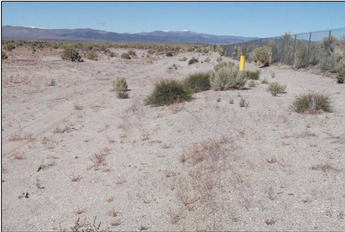
Plate 4-5. Landfill gas monitoring well GW-5 (view north).
