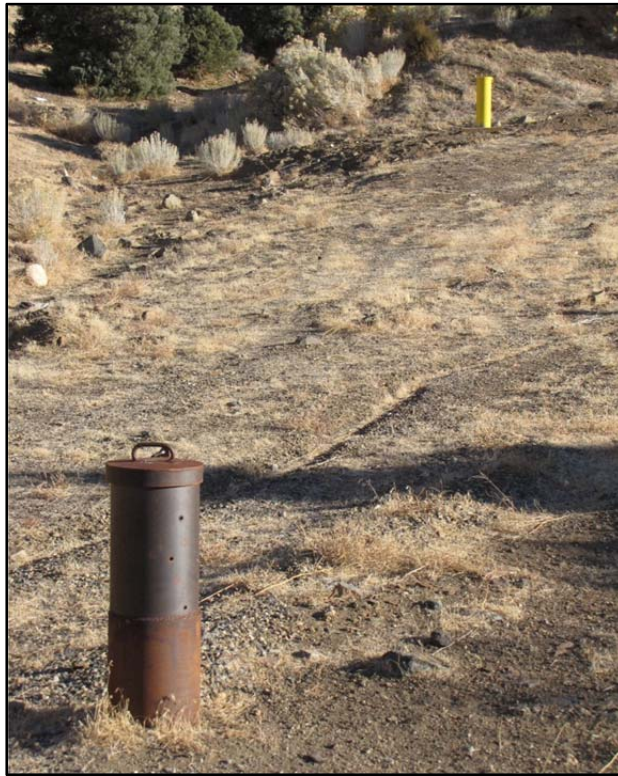
Plate 2-3. LFG monitoring well (background) from ground water monitoring well MW-2 (view north).
