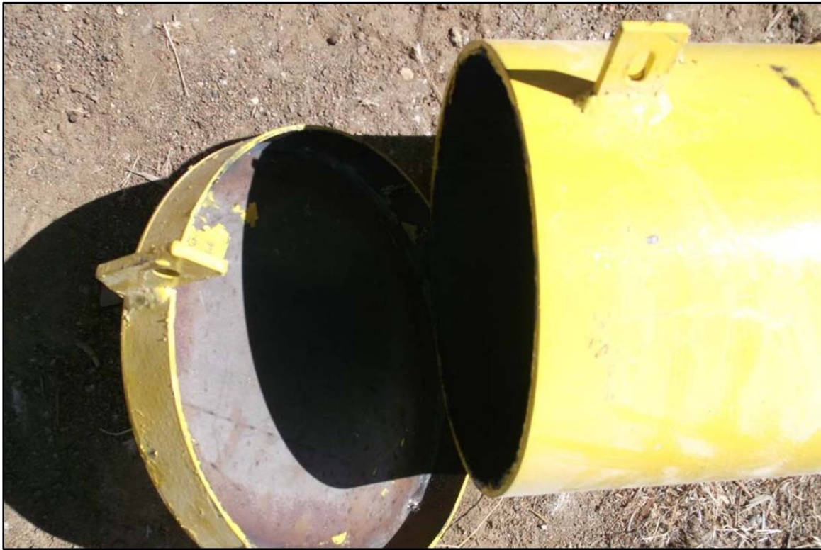
Plate C-5. Close-up of typical locking cap on painted steel surface completion monument.
