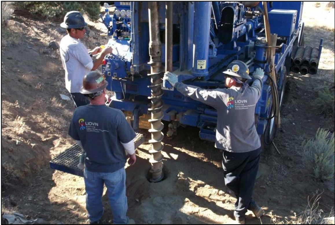
Plate C-3. Truck-mounted hollow-stem auger rig over borehole (Walker Landfill GW-1).
