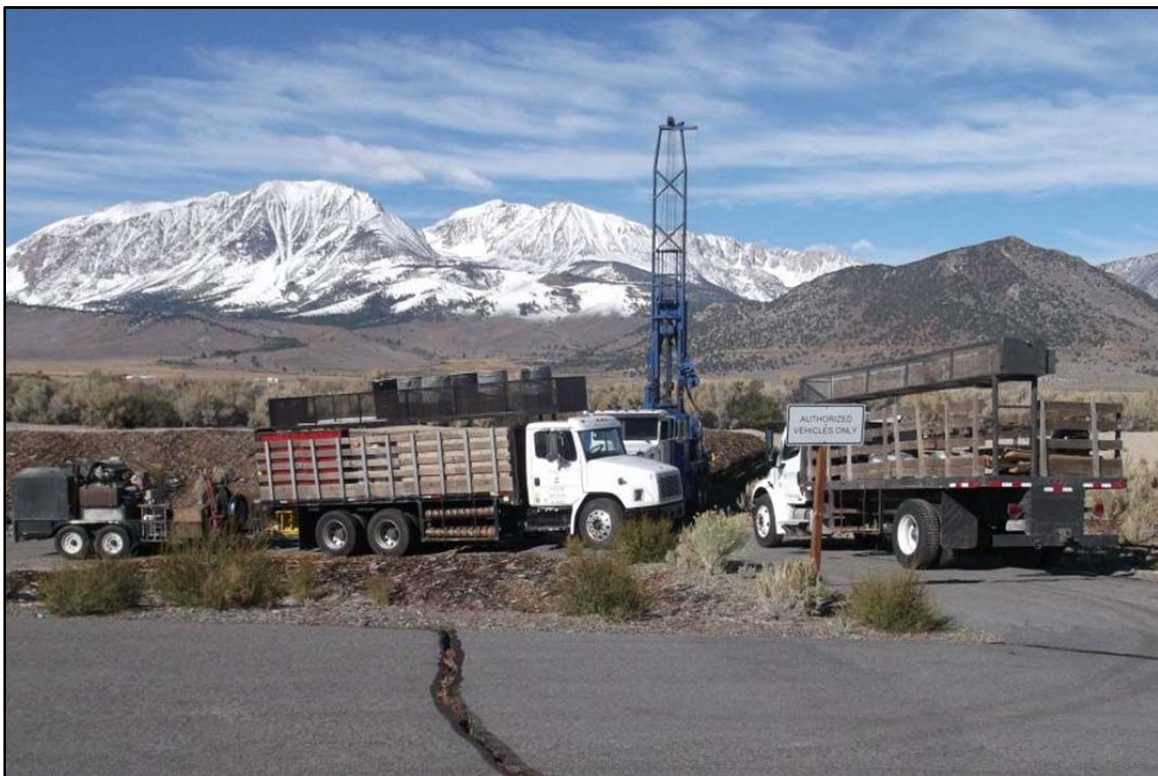
Plate C-2. Support trucks and equipment for drill rig (GW-1, view west).
