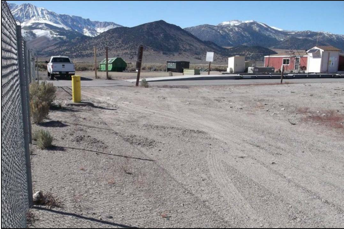
Plate C-15. Landfill gas monitoring well GW-7 at site entrance (view west).
