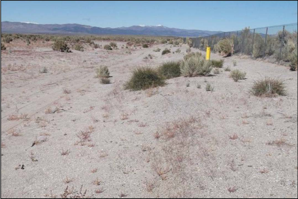
Plate C-13. Landfill gas monitoring well GW-5 (view north).
