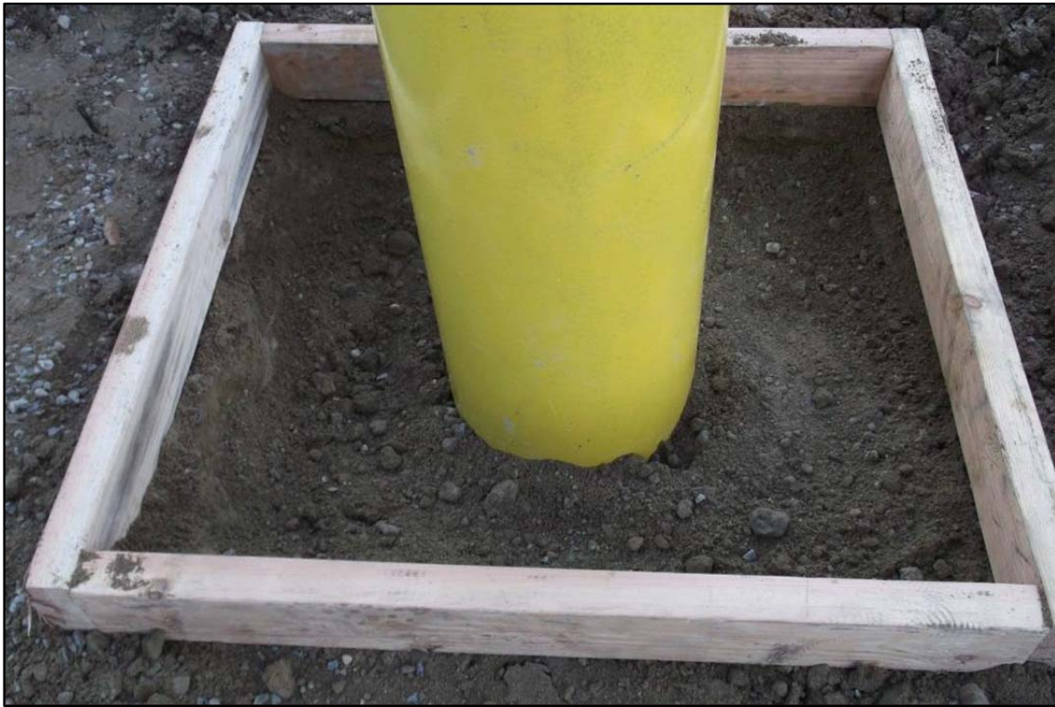
Plate C-7. Formwork and dug out base for surface completion concrete pad.
