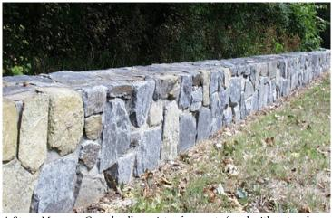
A Stone Masonry Guardwall consists of concrete faced with natural stone. Above: Caltrans guardwall in San Luis Obispo.
