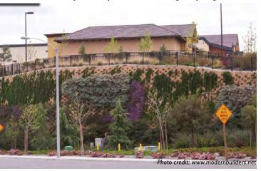
The VERDURA Living Retaining Wall system is a fully plantable block wall that is Caltrans approved.
