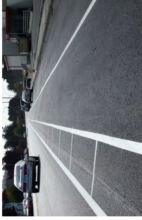
Buffered bike lanes add a 2-3 foot space to protect bicyclists from higher-speed traffic that would be present on a state highway.
