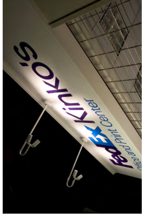
Sign lighting that faces down to reduce light pollution: B-K Lighting Twin SignStar Style A
