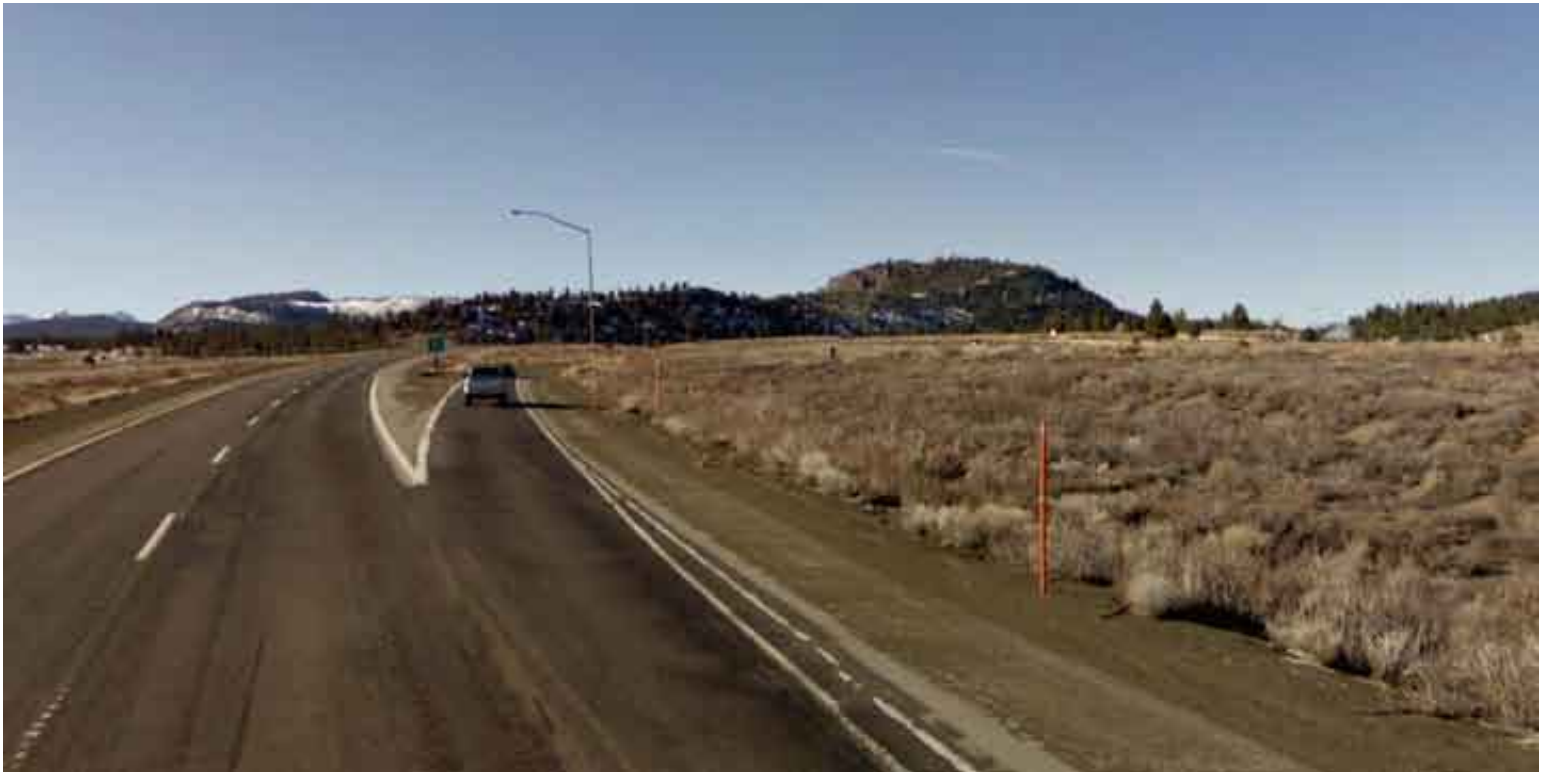
Mammoth Lakes Interchange Before Enhancements
