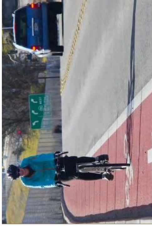
Colorized bicycle lanes are more visible to drivers; color can be integral to the asphalt mixture for increased durability.
