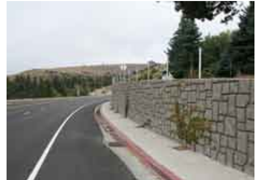
Lee Vining Streetscape with Enhanced Retaining Wall
