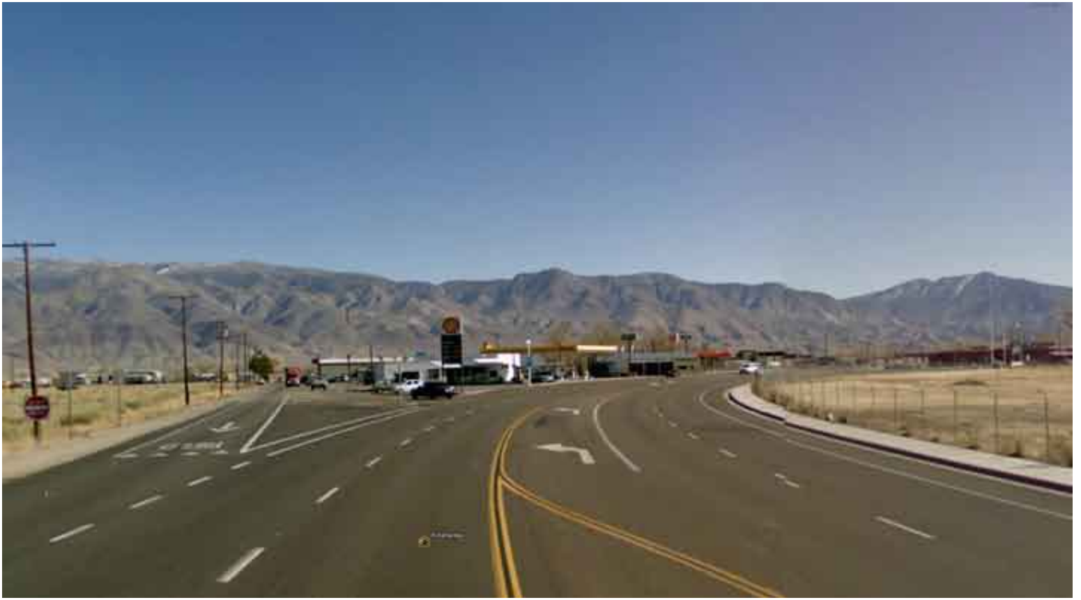
Bishop Entry at Wye Road Intersection Before Enhancements
