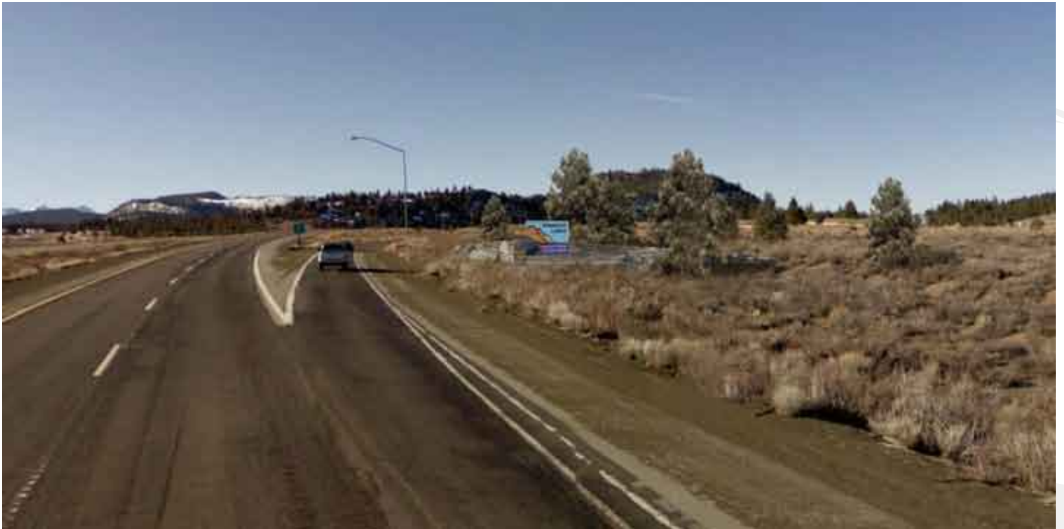
Mammoth Lakes Interchange After Enhancements
