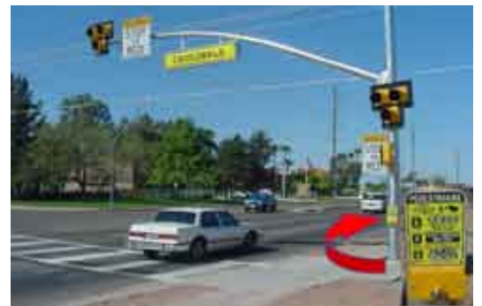
HAWK pedestrian signal – not currently allowed on Caltrans highways, but may be in the future.
