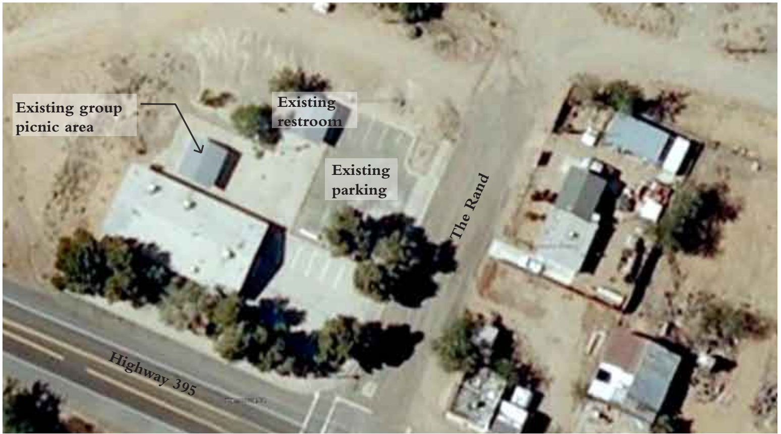
Johannesburg Park/Rest Area Before Enhancements
