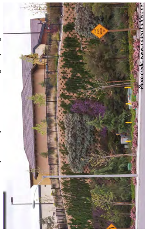
A structural, reinforced concrete retaining wall is covered by a sculptured veneer treatment and further softened with a railing and foliage.
