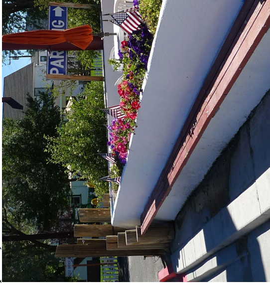
Wood fence is raised on a low masonry wall
