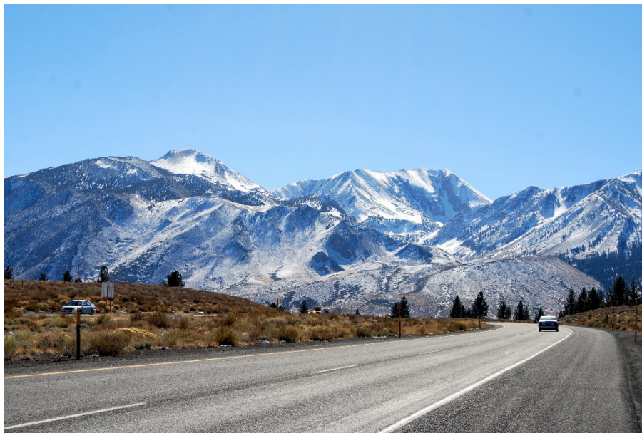
Figure 8: Section of Highway 395, near Mammoth Lakes
