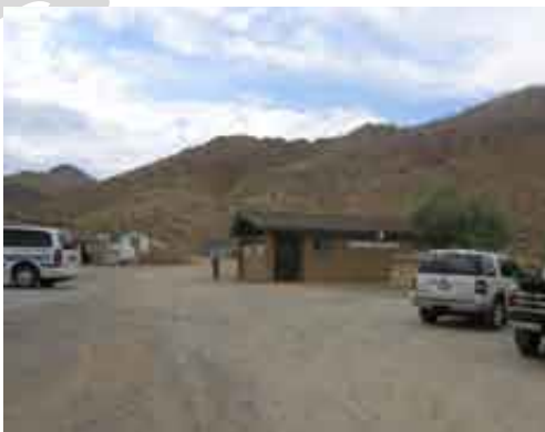
Public Restrooms at Park in Walker
