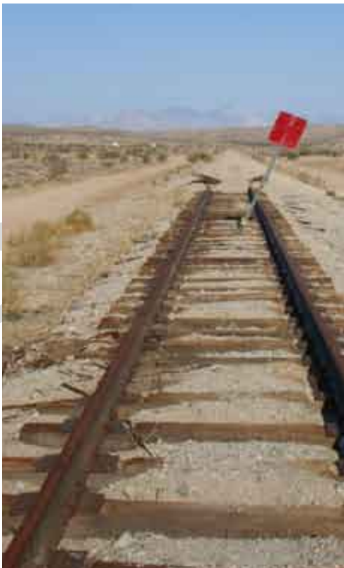
Old Rail Lines in Southern Inyo County
