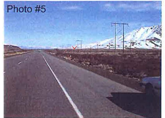
View from west along HWY 395
