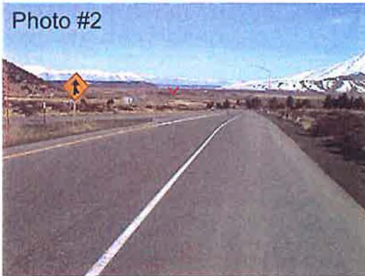
View from west at HWY 203 & 395
