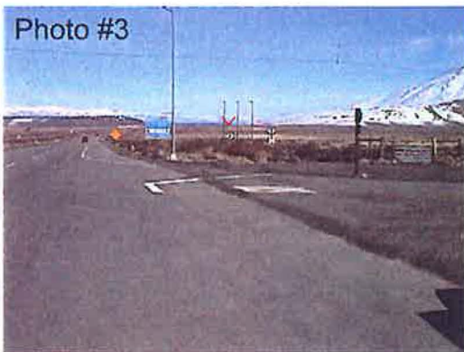
View from west at Mammoth Road & HWY 395
