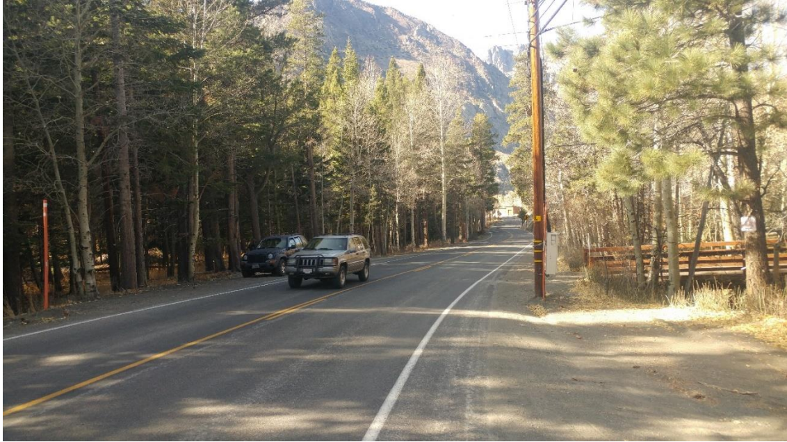
SR 158 at the intersection with Yost & Fern Lake Tailhead in the Down Canyon area. Absence of non-motorized connections between residential, commercial, and recreational destinations in this area unnecessarily encourages motorized travel.
