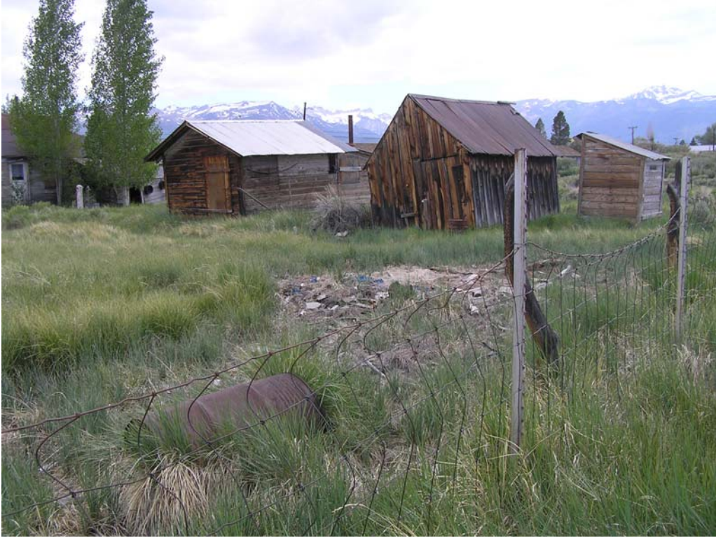
Overview of structures. View to the southwest.
