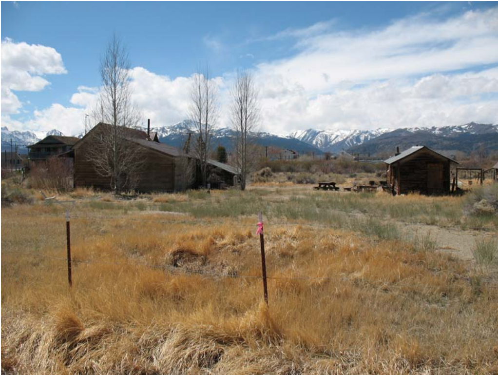
Overview of structures. View to the northwest.
