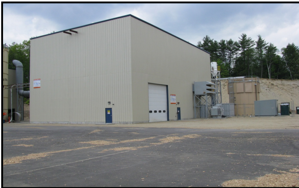
Exhibit 3-5: Zilkha Installation in New Hampshire
