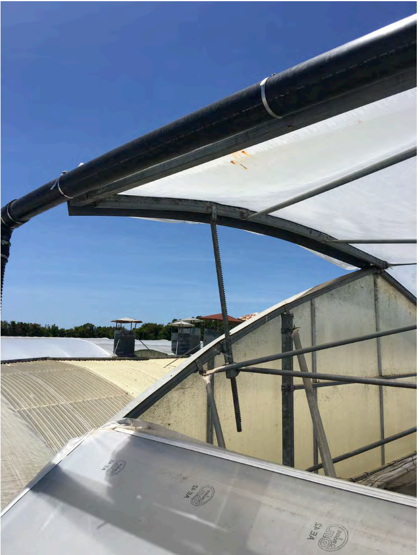
Vapor odor control system on ridge vent when vent is in open position
