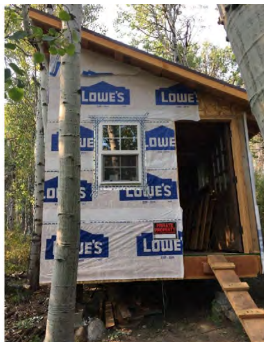
SITE PHOTO 1 – STORAGE SHED 09/30/2020
