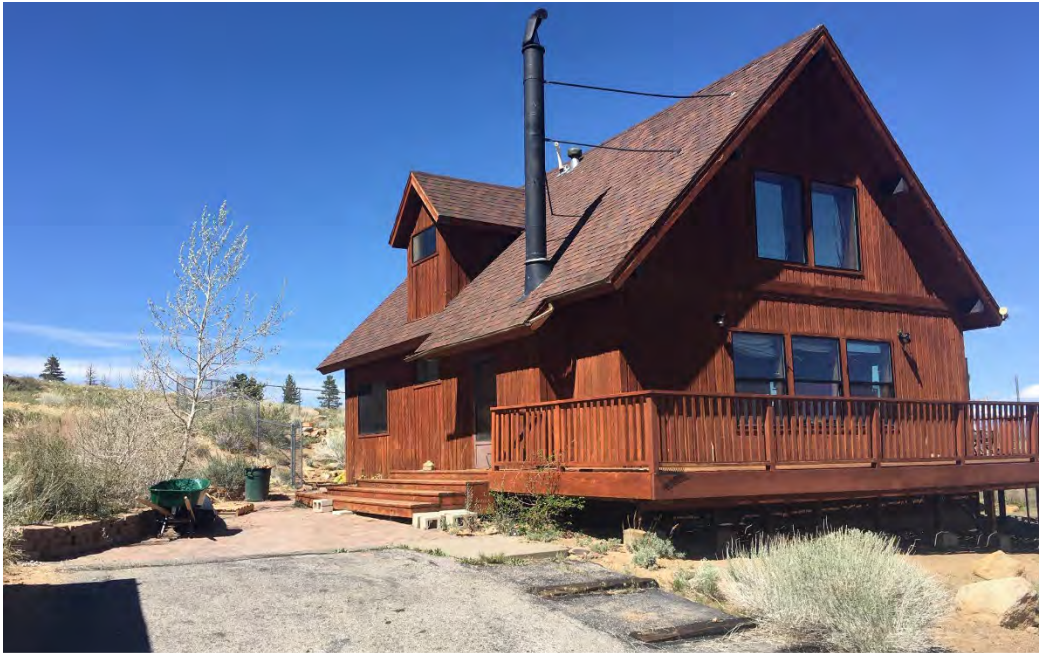
View of the existing residence from the top of the driveway.
