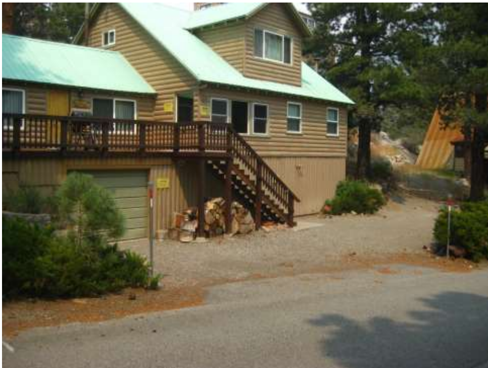
Figure 1: Front parking area
