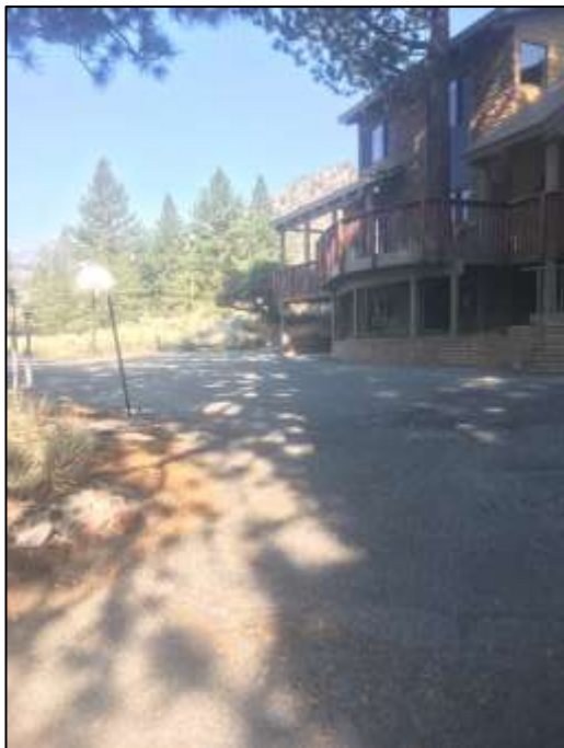
Figure 1: Front parking area
