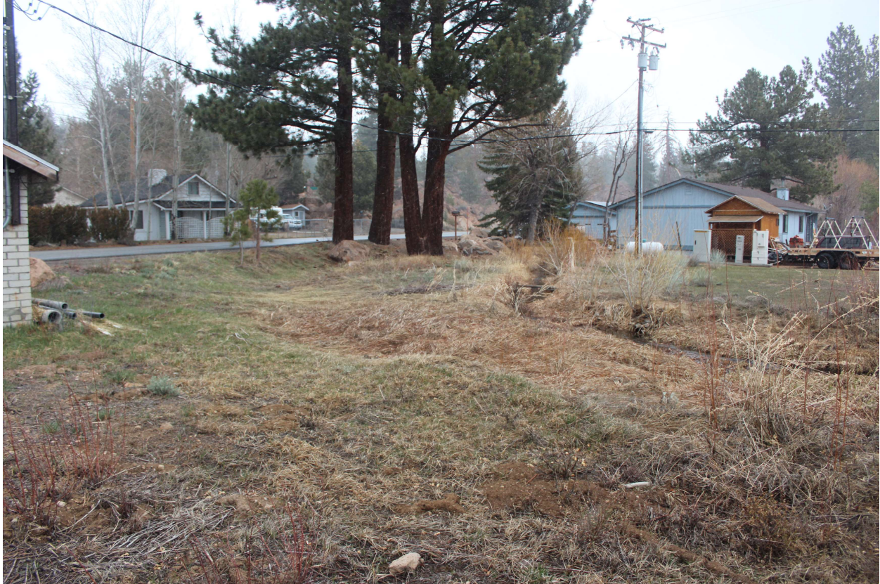
Rear of Building looking East – new SCE transformers will be on pole at property corner, out of frame in photo
