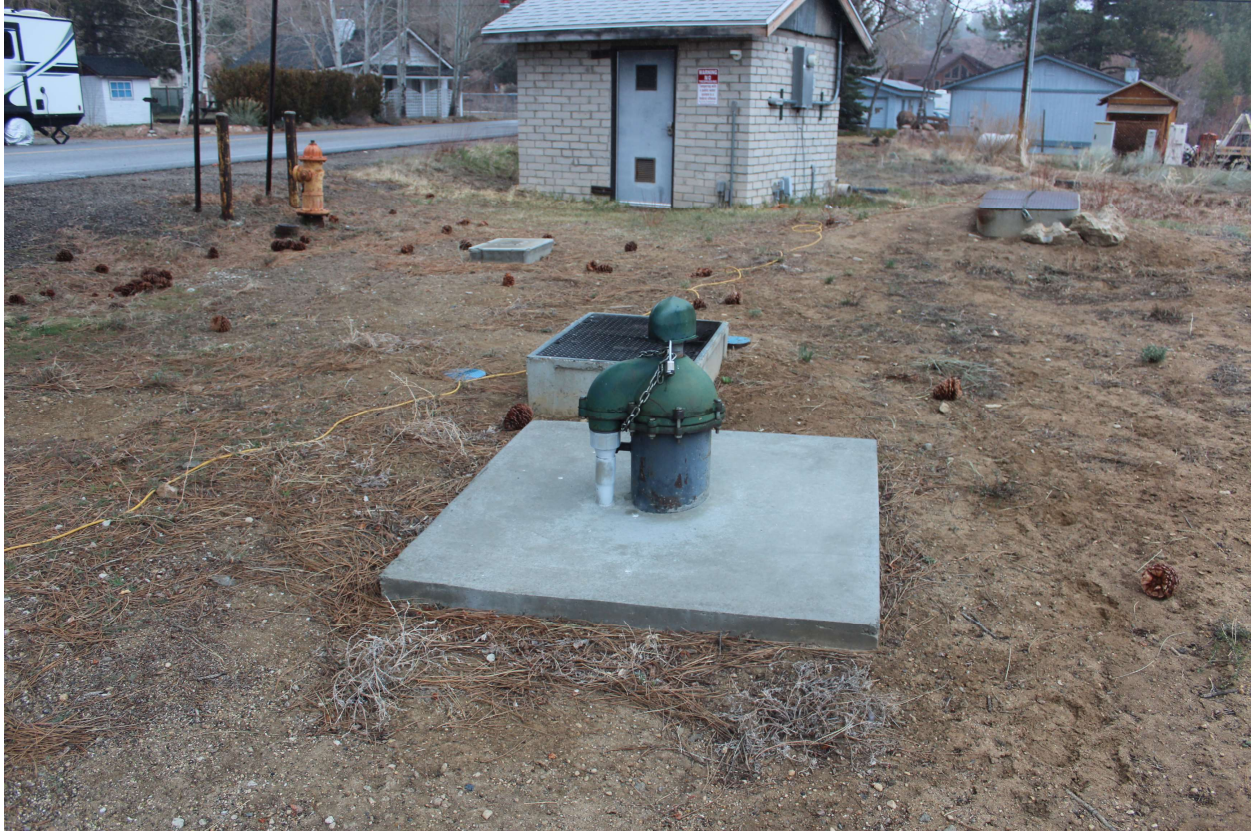
Rear of Building looking towards the East
