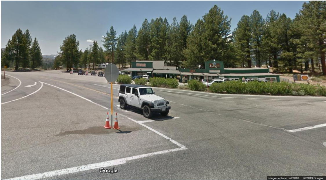
The southern entrance to the June Lake Loop (SR 158) at the June Lake Junction.
