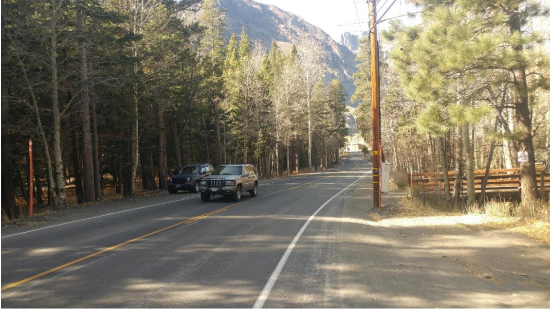
SR 158 at the intersection with Yost & Fern Lake Tailhead in the Down Canyon area. Absence of non-motorized connections between residential, commercial, and recreational destinations in this area unnecessarily encourages motorized travel.
