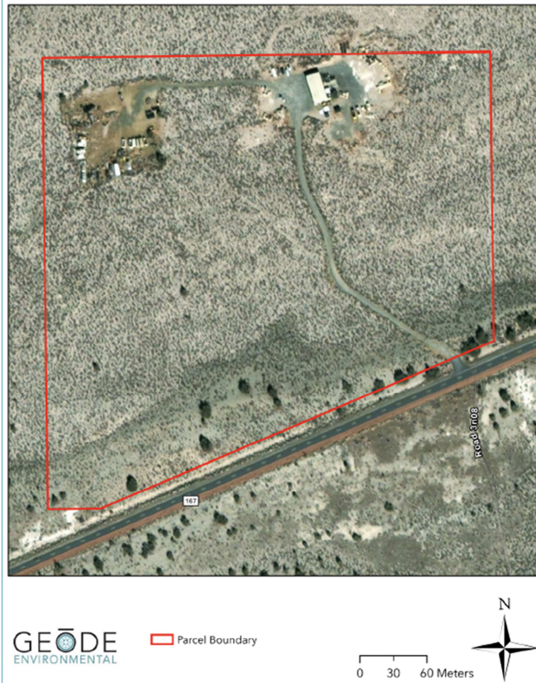
Figure 2: Existing site conditions
