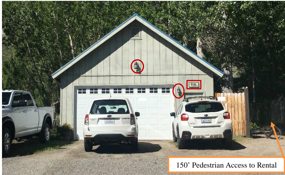
Existing exterior lighting and addressing at the property entrance.
