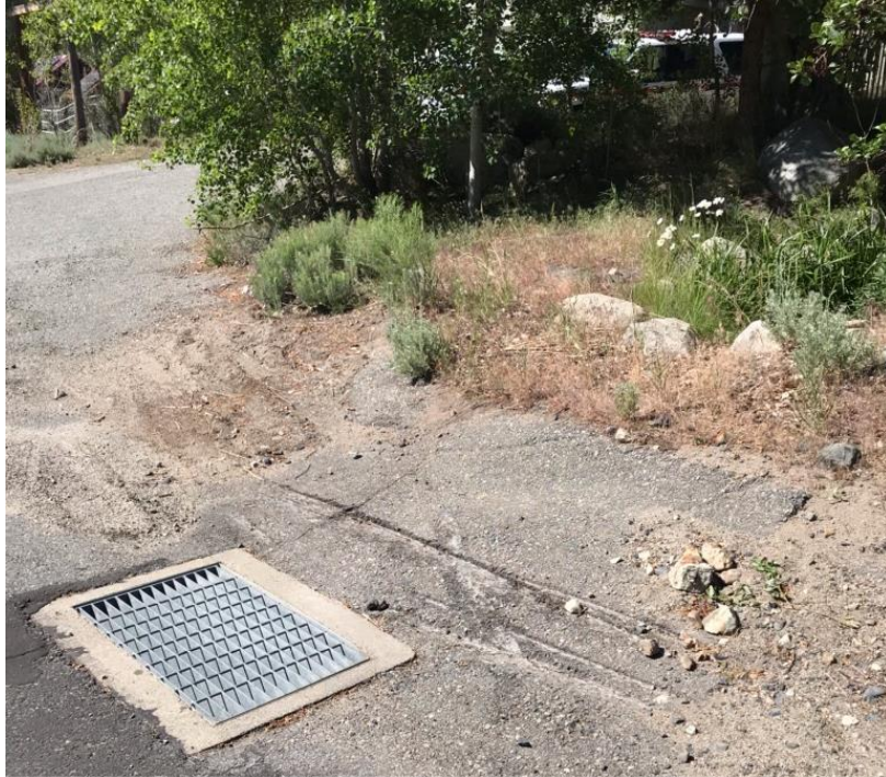
Possible emergency water draft point #2, a culvert located just outside of the project property line.
