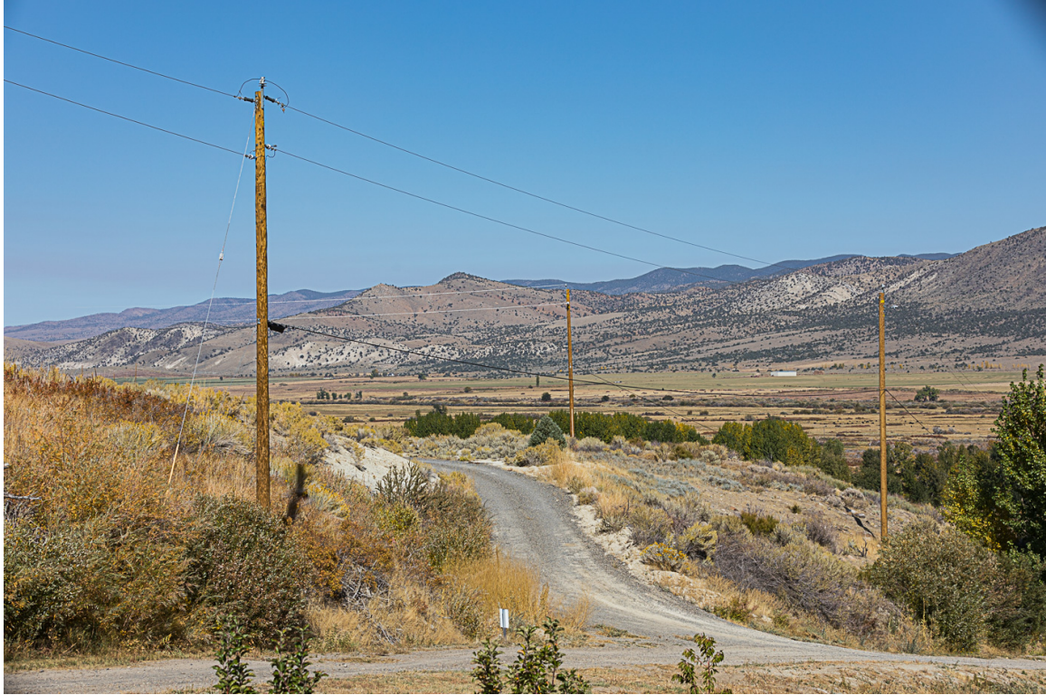
Figure 3 Drive to #162. Too steep. All new poles
