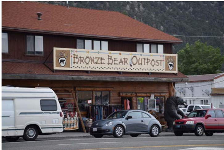
Wood siding with log lintels
