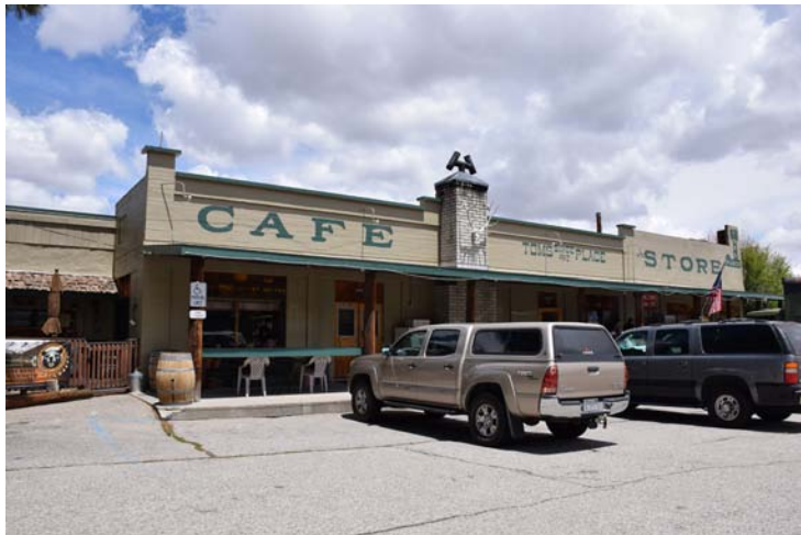
Storefront with parapet and canopy
