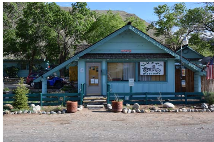
Mid-century roof frame with wood siding
