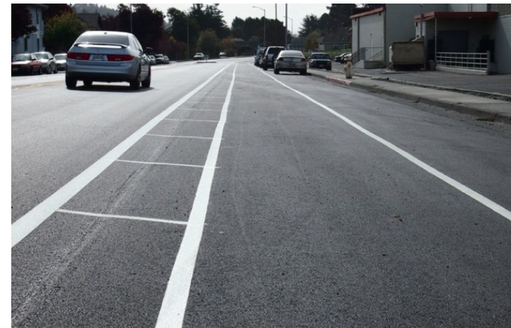
Buffered bike lanes add a 2-3 foot space to protect bicyclists from higher-speed traffic that would be present on a state highway.
