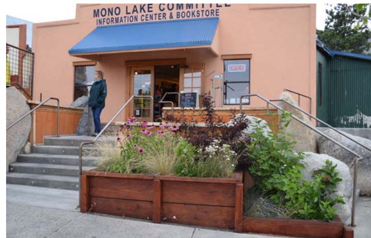
A terrace in Lee Vining provides public space and space for landscaping.
