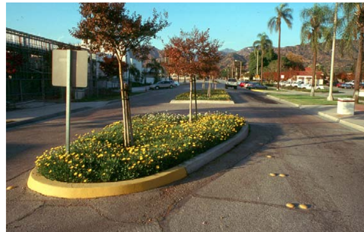
Median islands make the travel lane visually seem tighter, which can help reduce speeds and make a community more walkable.
