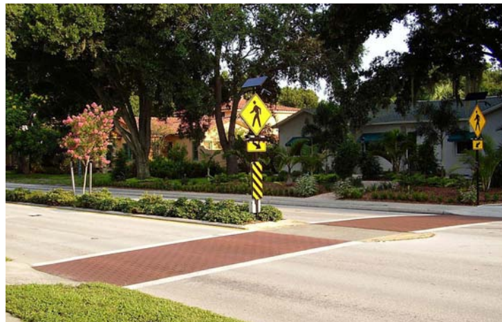
Stamped concrete has the appearance of brick; this both provides a color for visibility and a tactile reminder to drivers to slow down.
