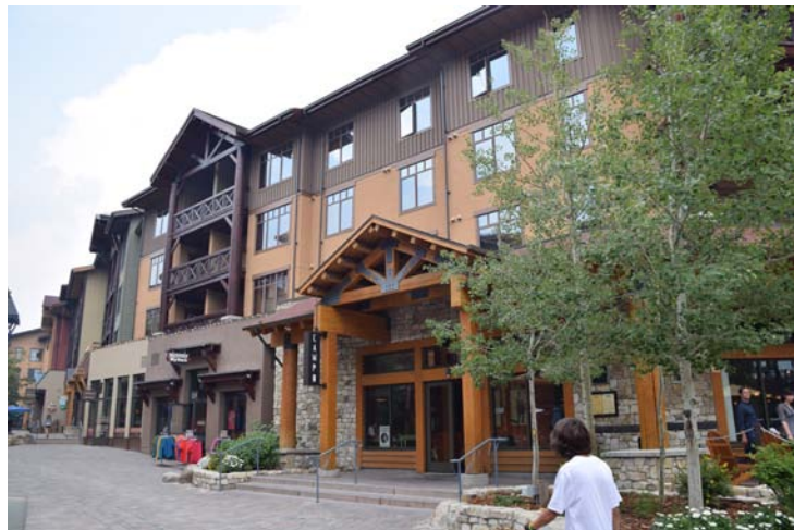
Stoop of Heavy timber construction
