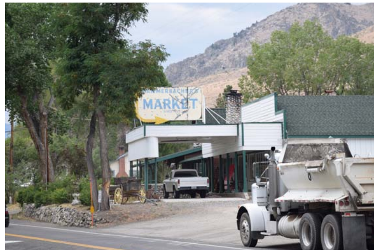
Historic drive-through with retaining wall
