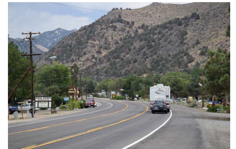
Wide right-of-way encourages high speeds.
