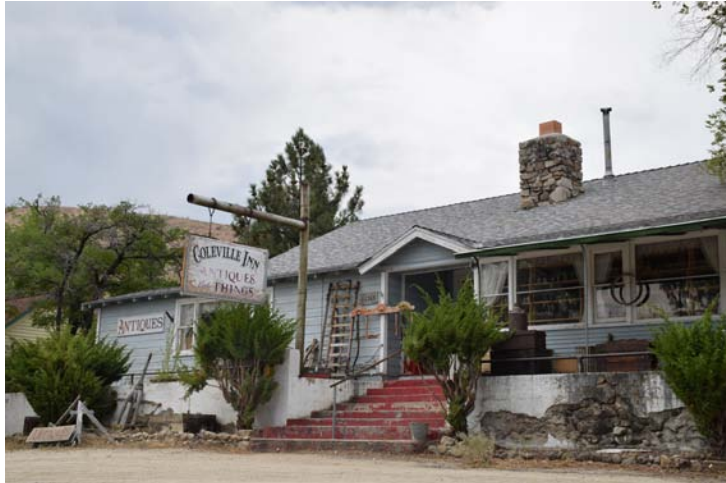
Building with recessed stoop and wood siding
