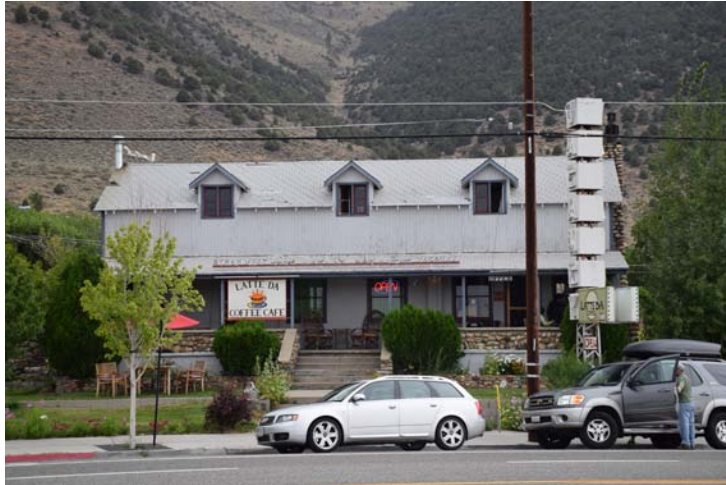
Metal roof with dormers and a deep porch
