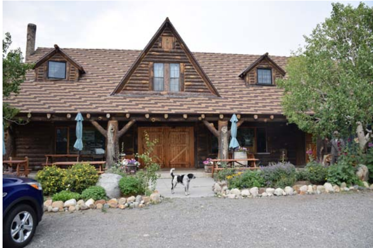
Wood siding and tree trunks for columns
