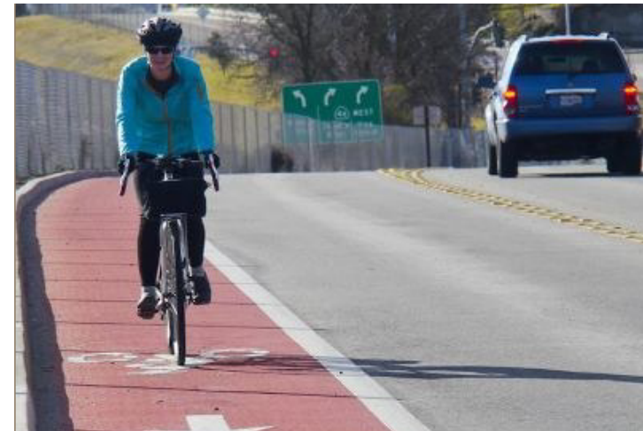
Colorized bicycle lanes are more visible to drivers; color can be integral to the asphalt mixture for increased durability.
