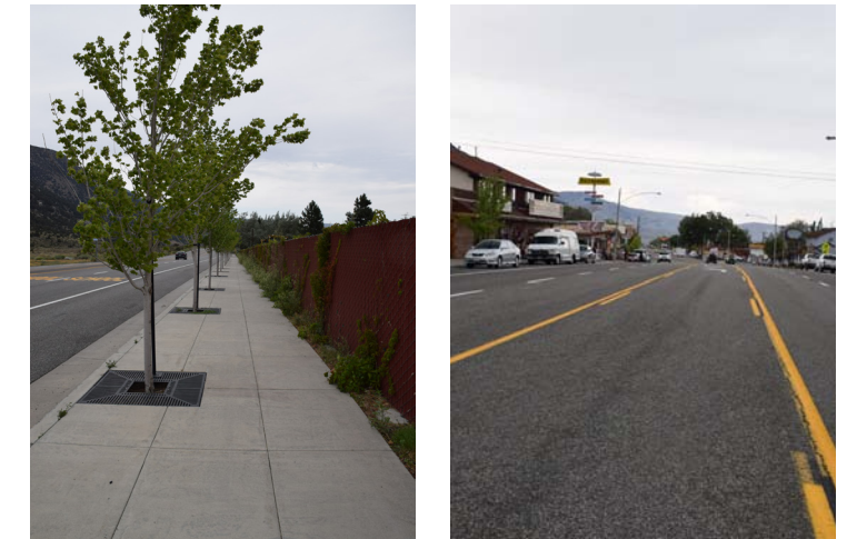
Recent sidewalk improvements; wide 5-lane right-of-way with no crosswalks
